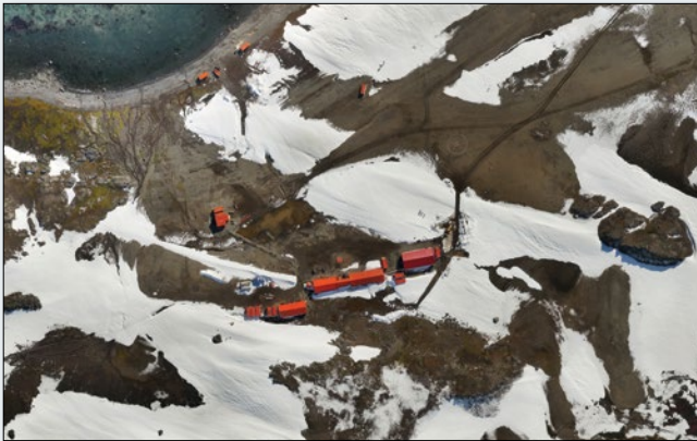
Prepared using the Trimble Business Center Photogrammetry Module, this orthophoto of the Maldonado Base was taken by the UX5 from an altitude of 100 m (330 ft)
